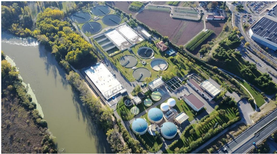
Figure 4. The Logroño - Bajo Iregua WWTP in the Northeastern limit of Logroño
